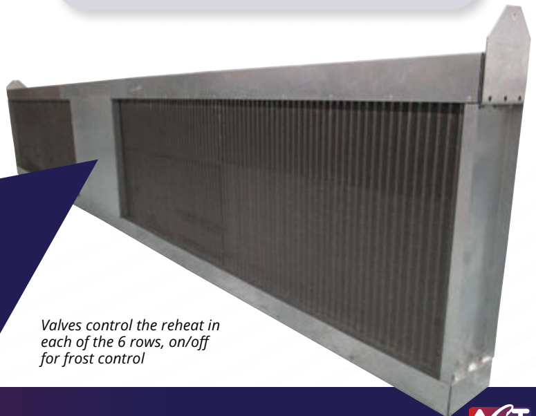
SPLIT LOOP THERMOSYPHON: 2 PIPES PER ROW
