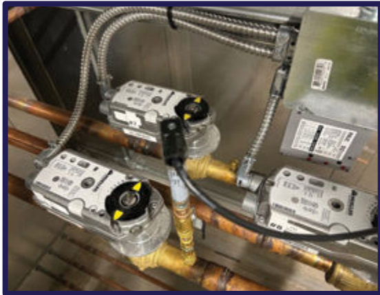
Example of heat transfer capacity control valves
