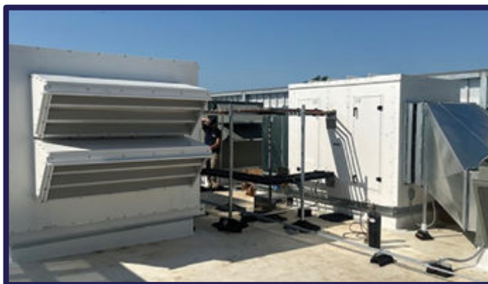
Above: Large WAHX systems can be installed in sections.
