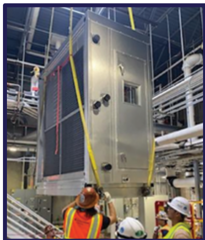
Above: Large WAHX systems can be installed in sections.
