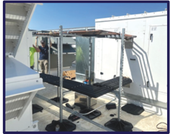
Air-to-Air Split loop energy transfer between 15 foot separated exhaust and supply air AHU's. Precool and preheat incoming air from exhaust AHU.
