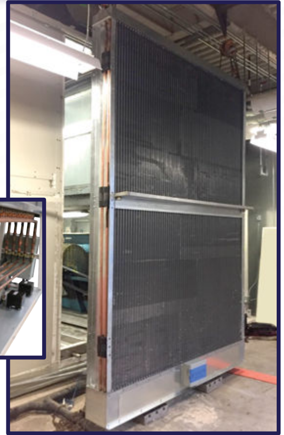
Above: Half of a large AAHX unit being installed.
