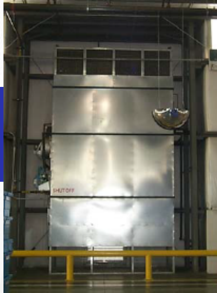
Figure 1: IFA-300/200 w/ 60 Tons of Cooling & 2,000 MBH of Heating
