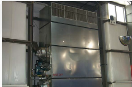
Figure 2: Indirect Fired HX w/ Power Burner & Exhaust Flue
