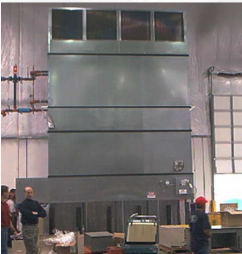
Figure 3: IF-A-600-C Air Turnover Unit 100 Tons/58,000 cfm
