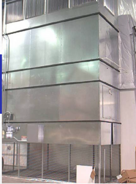
Figure 1: IFA-600-C Air Turnover Unit 100 Tons/ 58,000 cfm
