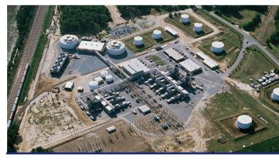
**The Butler-Warner Power Plant** in North Carolina - the world's largest thermal energy storage (TES) project to date - depends on half-a-million feet of stainless steel tubing in 112 Heatcraft custom coils to help cool air used in generating electricity. The 112 cleanable Heatcraft coils were custom-made, delivered and installed one week ahead of schedule.
